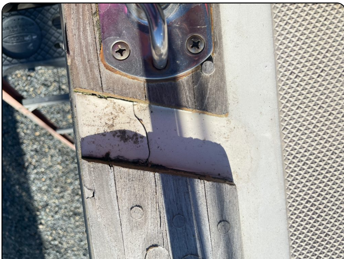
Crack in cap rail and teak toe rail
