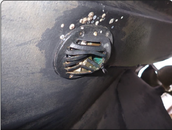
Replace the scoop at the next haul out
