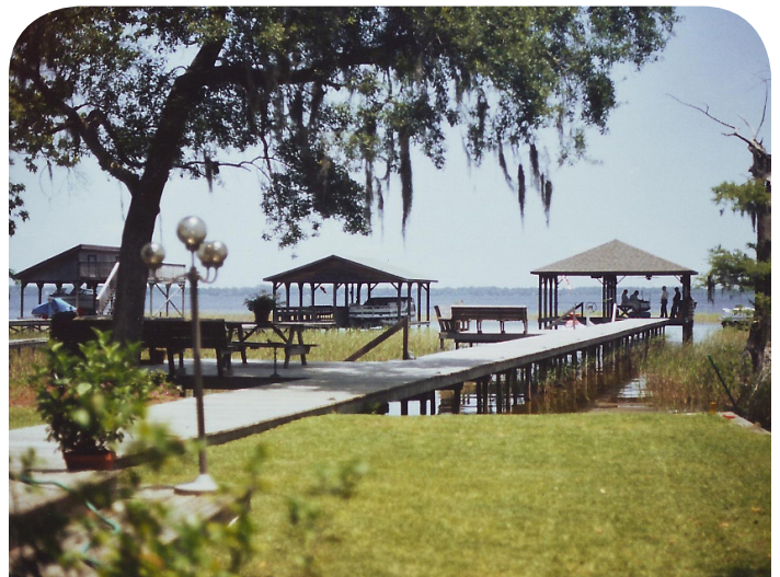
Photo 1. The boat dock on the far right is where the accident occurred. The wiring to the dock is routed on the opposite side of the walkway.
