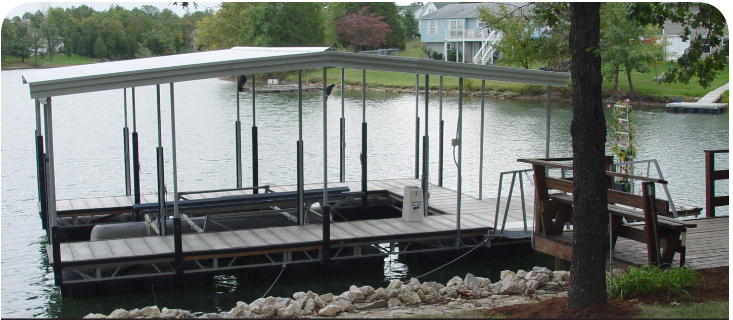
Photo 1. After conducting a forensic investigation and analysis, the electrical engineering expert on this case determined that the dock wiring was not the cause of electric currents in the lake water.
