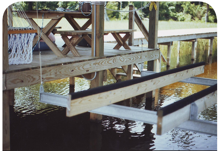
Photo 2. This image is of the boat lift assembly that was energized, with the metal rails visible, attached to the metal wires.
